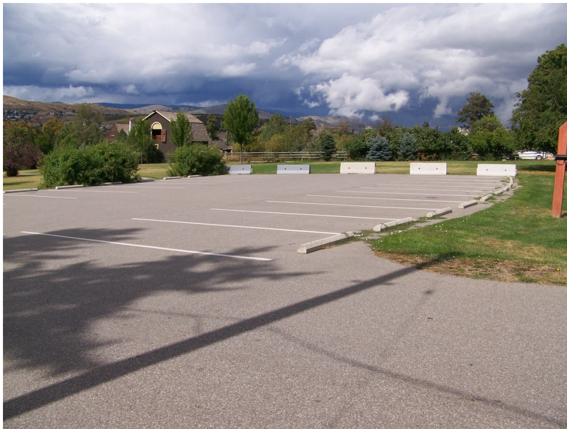
Photo 4: Sovereign Park MFV Parking Area
